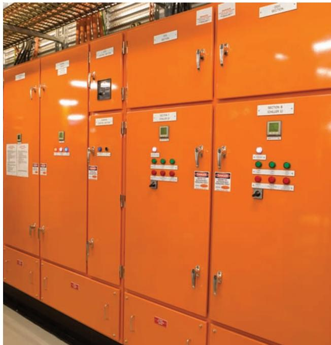
Variable speed drives (left) and custom built mechanical services switchboard (right) are part of a trigeneration system in Australia.
