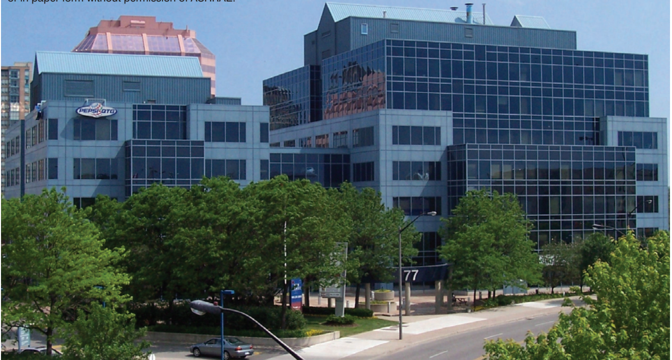
Photo 1: The City Centre complex in the Toronto greater metropolitan area uses a Web-based BAS.
