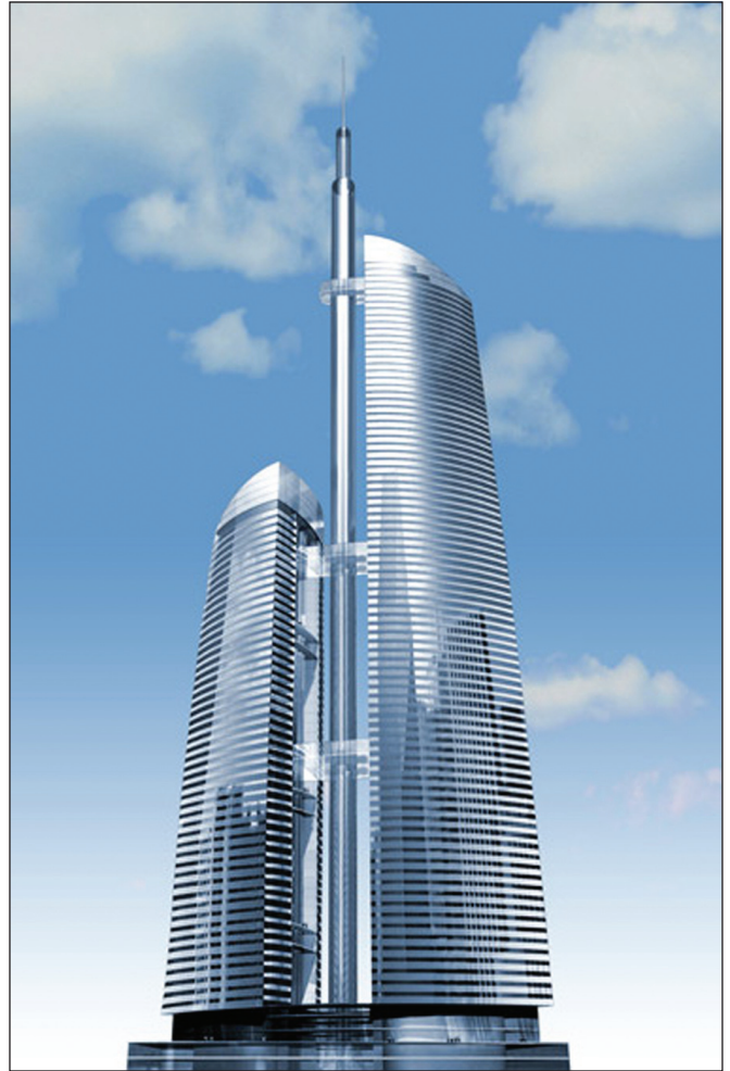
The Federation Tower in Russia is designed to be the tallest building in Europe when completed in 2008. BACnet was chosen to give the building owner future flexibility as the rest of the project is being built.
