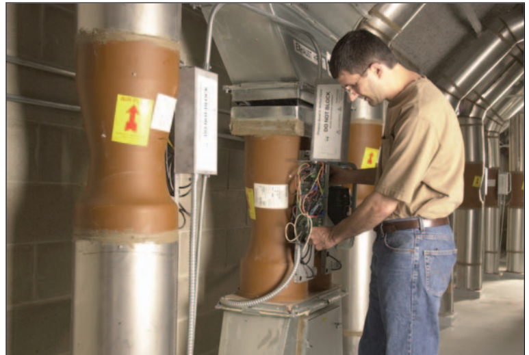
Upper left: BACnet enables the integration of 88 laboratory fume hoods, such as this one with the building automation system. Upper right: the Science Laboratory Center opened for classes in fall 2004. Lower left: Facility staff can monitor and control the laboratory fume hood system from a workstation in its control room across campus. Lower right: The fume hood valves and controls are located in a penthouse above the laboratory classrooms.
